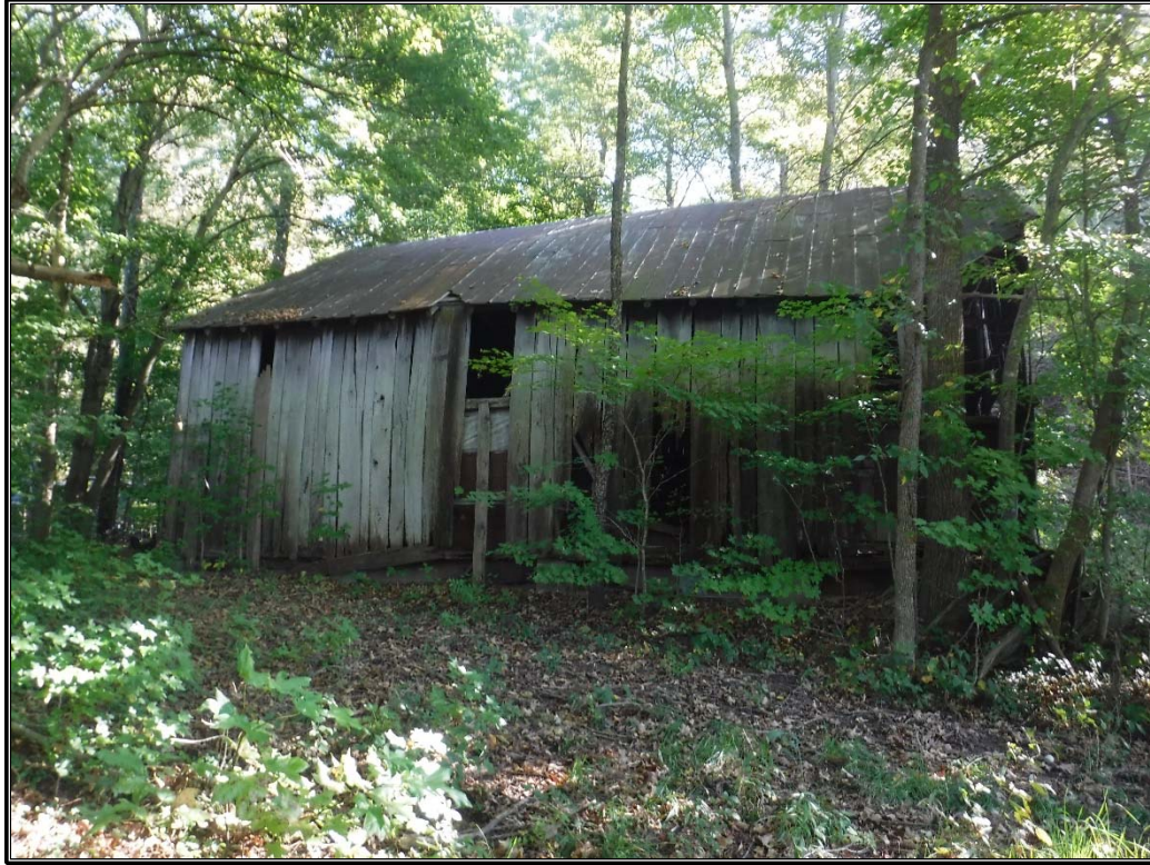
Figure 17. Barn at MS 7 area, facing east.
