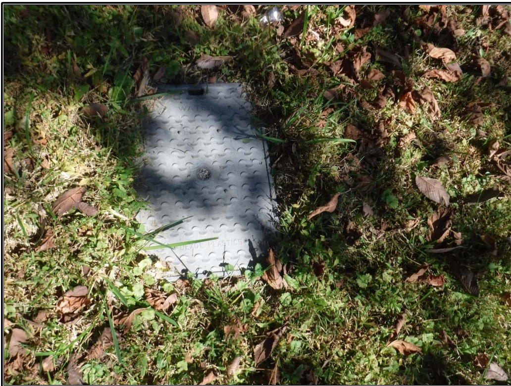
Figure 7. Underground utility, facing east.
